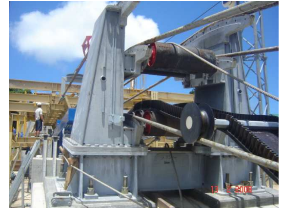
Simberi Gold conveyor under construction
