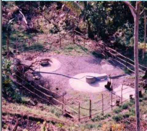
Sissano tsunami disaster rehabilitation center's water supply. hand dug shallow well was constructed under close supervision of the branch for Caritas PNG.
