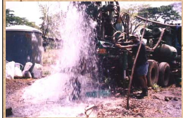
Developing a successful borehole drilled for PNG Waterboard at the KB well-field in Alotau for the town water supply. Groundwater is used to supplement the surface water scheme that sometimes runs dry during prolonged dry seasons.
